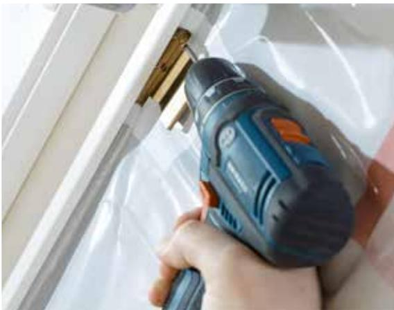
**3.** Install mounting clips to skylight drywall groove.
