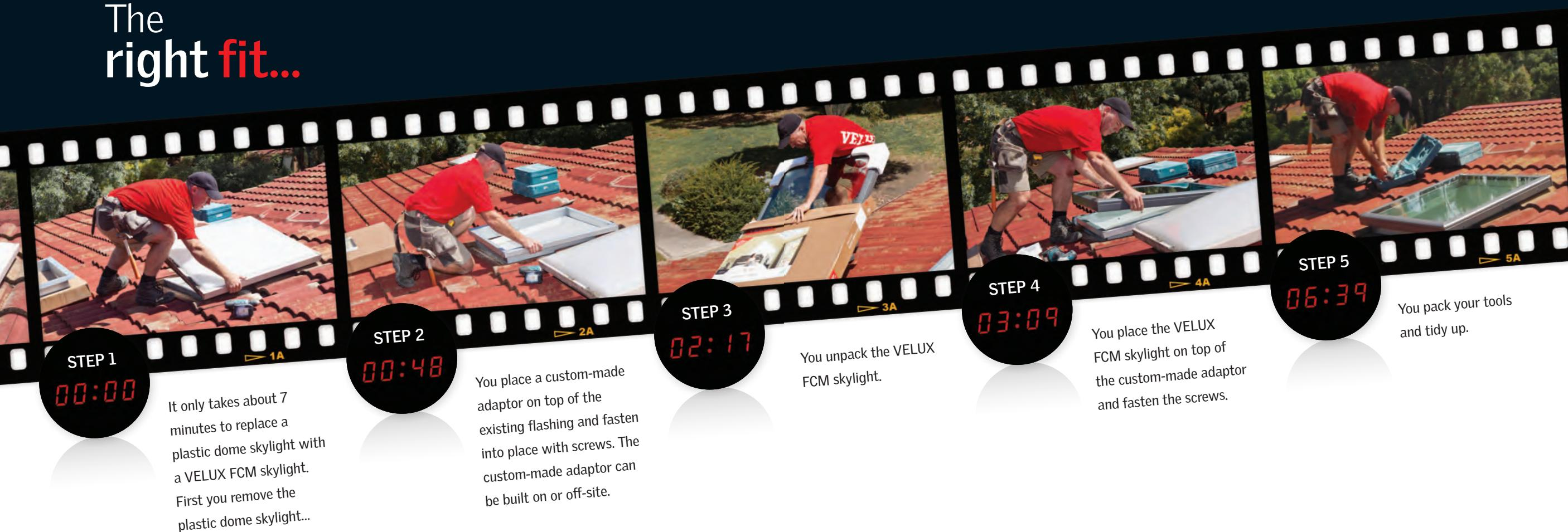
The trial installation was performed by an independent VELUX installer in Melbourne on 24th January 2011, into a tiled roof at approx 15° pitch. Please contact VELUX for a copy of the video showing the actual installation.
