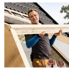
3 Middle trimmer • laminated pinewood • customised, no adjustments
