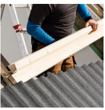
1 Bottom trimmer • laminated pinewood • customised, no adjustments
