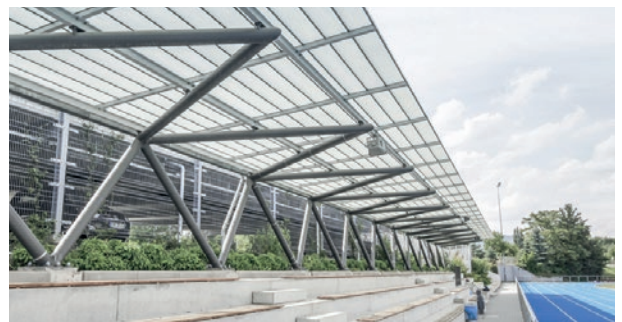
Roofing of a sports tribune with GRILLODUR®
