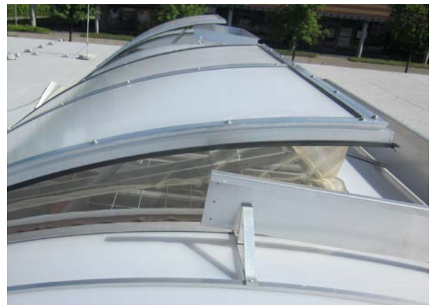
Continuous rooflight flap in ventilation position with insect screen system
