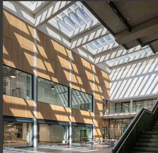
to any desired position, whilst the smoke venting modules are controlled as part of the building management solution. For the installed VELUX Northlight solution, both the blinds and comfort venting modules are controlled by the VELUX INTEGRA® system.
