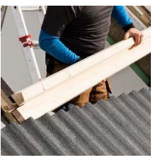
1 Bottom trimmer • laminated pinewood • customised, no adjustments
