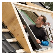
5 Frame insulation collar BDX • shaped polyethylene in a steel frame • easy and effective insulation around the frame
