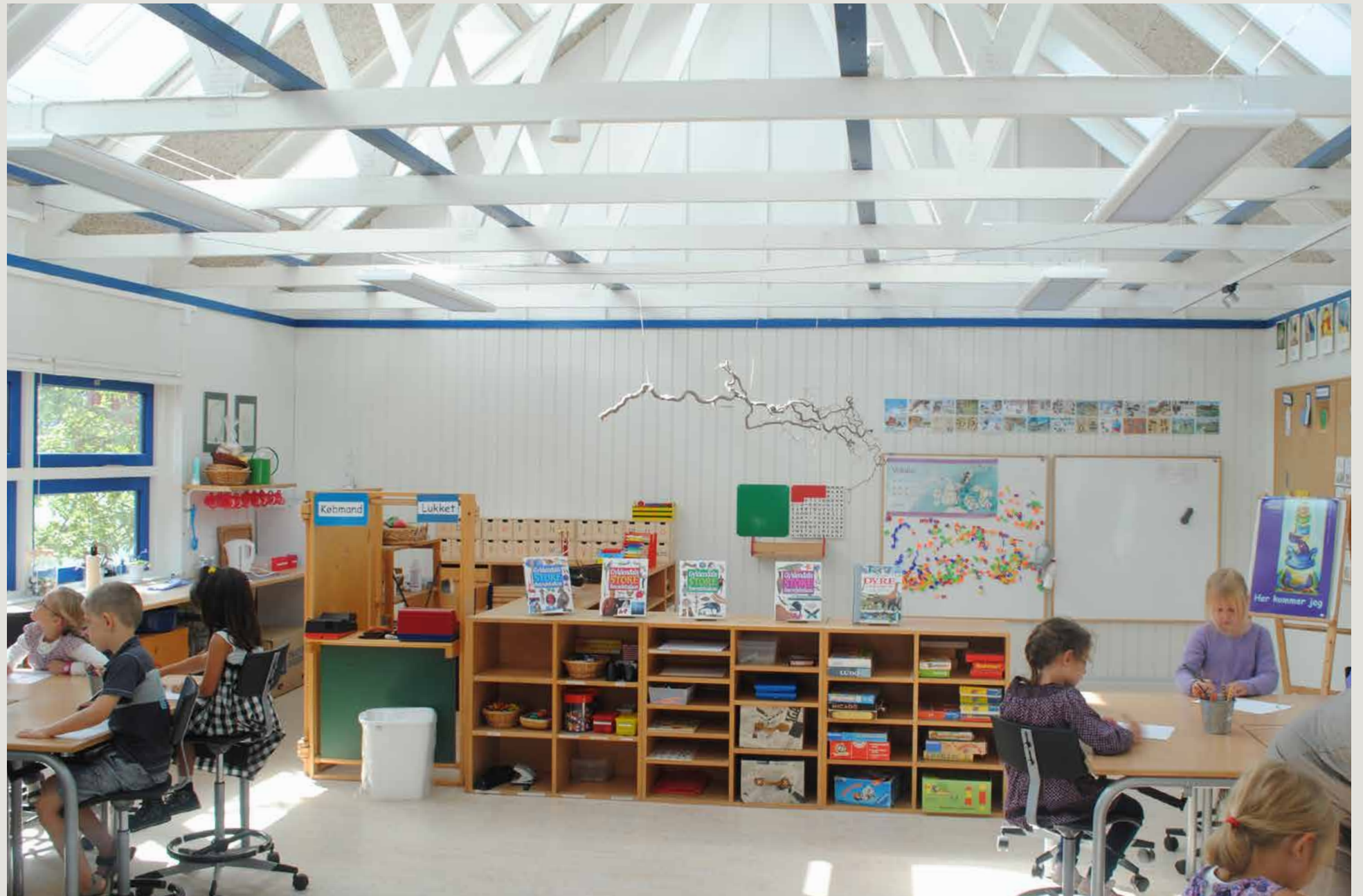
After renovation and installation of VELUX roof windows.
